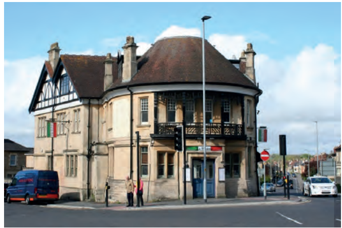
Fig 3.8: The former Little George is a local landmark at the road junction, particularly when approaching from Langley Road, though its less attractive rear elevation is prominent approaching from Park Lane on the one-way system. Highway infrastructure also compromises the setting of this listed building.
