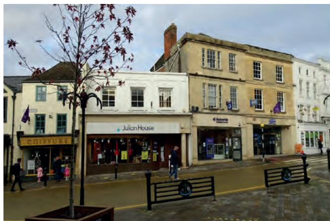
Fig 14.4: These three buildings in the centre (originally all building societies) now have modern stone shopfronts, all partly recessed. Apart from No. 51-52 fascia lettering is subtle, and overall does not jar with the historic character.
