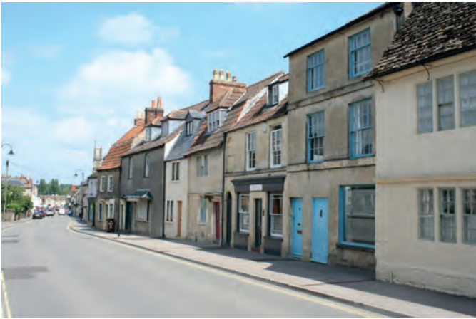
Fig 17.5: No. 30 (centre) makes a positive contribution to the character of the area. To the right is a former shop converted to residential. Like a number of such buildings in the street it retains its shop window.
