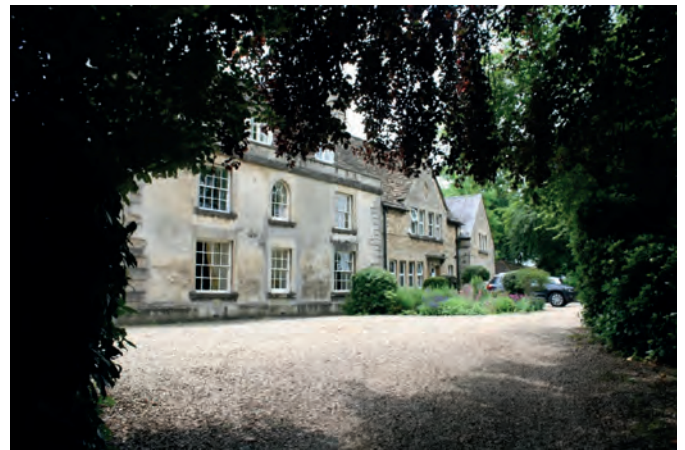
Fig 9.5: The fine frontage of the listed Lowden Manor in its secluded cul-de-sac. Modern top-hung replacement windows (right) are an intrusive and inappropriate feature.
