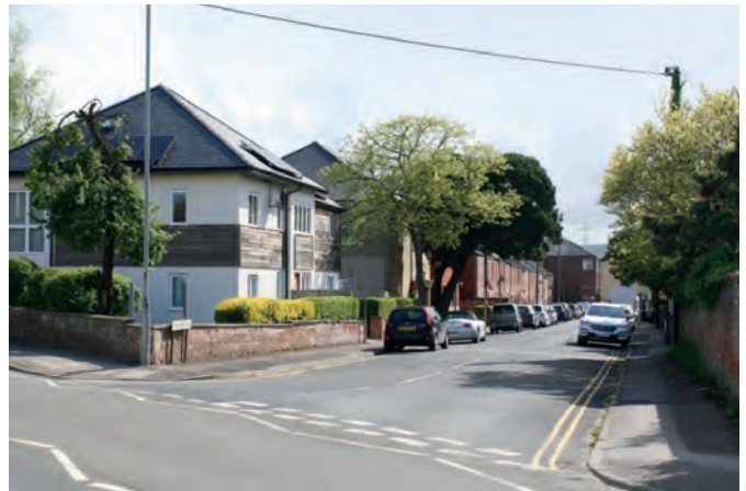
Fig 5.4: This modern block of four flats turns the corner well, and is a positive insertion into the street scene.
