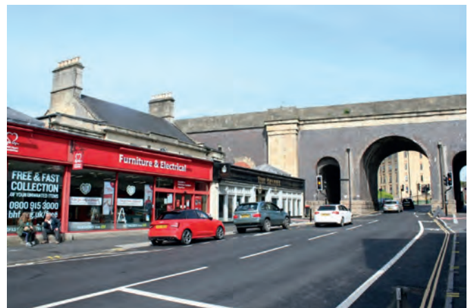
Fig 7.9: The improvement in the design of shopfronts, plus the restoration of the viaduct, have been welcome. It is still a shame that the quality of the Grade 2 listed 'Brotherhood' ex railway works office is only really able to be appreciated from inside the Brunel pub.
