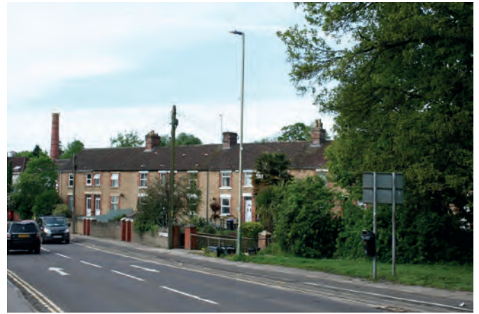
Fig 6.4: Providence Terrace is an attractive row of houses set back from the traffic. Replacement windows and doors have undermined the visual coherence of the terrace.
