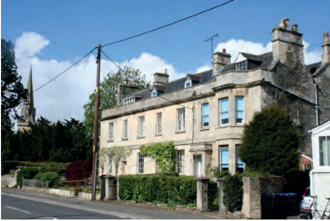
Fig 5.3: The fine entry into the town from Langley Road is enriched by this lovely terrace of early 19 th Century houses. Reinstatement of railings would improve them still further.
