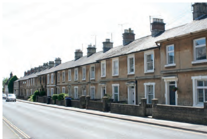
Fig 1.2: This fine listed terrace was built by Rowland Brotherhood for workers at his factory on Foundry Lane and many original features, such as sash windows, remain. Note the loss of a chimney stack, painting of stone window surrounds and the loss of railings for walls, all features detrimental to the character and overall unity of the terrace.
