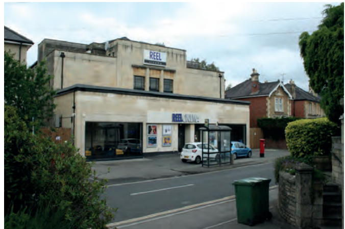
Fig 1.7: The refurbished Reel Cinema is a fine Art Deco building.
