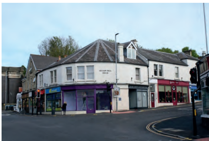
Fig 7.11: This parade of shops has recently seen some improvements although shopfronts could be further improved. Stricter advertisement controls could help secure improvements to the appearance of these shops. Replacement windows and painting of stonework at upper floors have diluted the character of these otherwise simple but attractive buildings.
