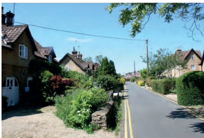
Fig 5.2: The Hamlet is an exceptionally picturesque lane with a rural ambience to it. Overhead cables and yellow lines are particularly dominant and intrusive features. Their removal would improve the character and setting of the street and listed buildings immeasurably.
