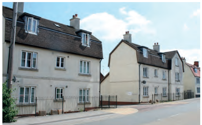
Fig 18.2: Nos. 1-9 Royal Oak Close located adjacent to the listed former Royal Oak pub, though is somewhat chunky in appearance. Unfortunately lack of attention to detail make these rather bland buildings.
