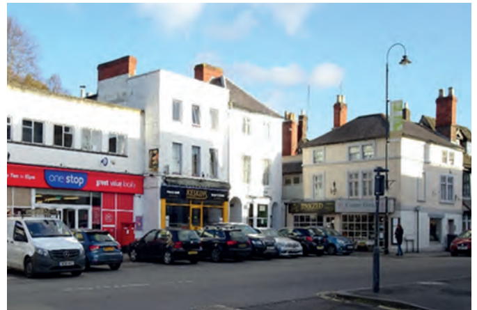
Fig 14.10: These once fine buildings have acquired a number of unsympathetic alterations over time, notably painting, advertising, modern shopfronts and replacement windows that have severely compromised their character and contribute to the generally unattractive appearance of this part of the Market Place. However No. 25 on the right has been sensitively refurbished.
