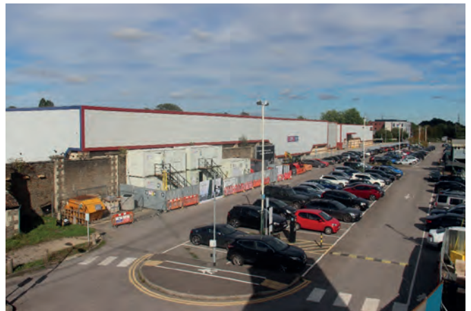
Fig 4.1: The monolithic blank rear façade of the Hathaway Retail Park is a particularly unattractive feature. It isolates the station from the north of the town and blocks views of the Grade II* listed St. Paul's Church.
