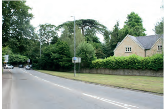
Fig 9.1: The approach from Bath Road is distinctive due to the landmarks of the fine Cedar tree and the laundry chimney.
