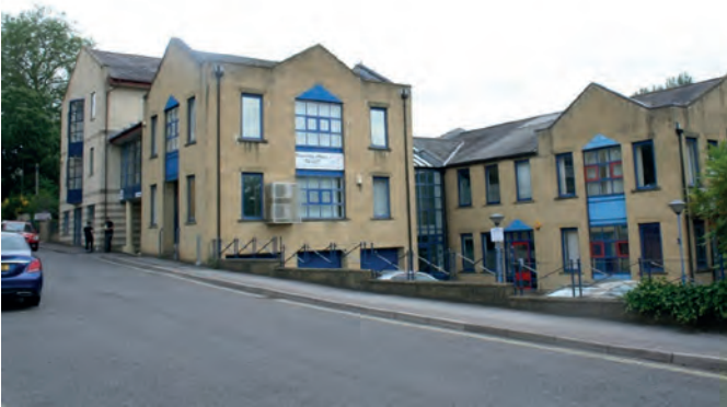
Fig 8.3: The main office development at Avon Reach is of bland blockwork and its form relates poorly to the street, making the car park a prominent feature. The office block furthest to the left relates better to the street and resolves the parking arrangement far more satisfactorily.
