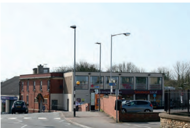
Fig 4.2: The old Post Office sorting office, where the concrete frame of the 20 th Century part has been incorporated into the Sainsbury's store.
