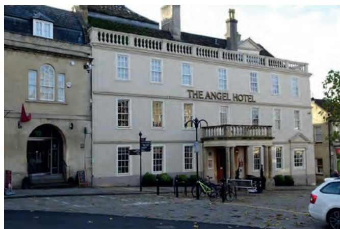
Fig 14.13: The Angel Hotel is one of the most important and imposing buildings in the Market Place. It is unfortunate that the stone dressings on the building have been repeatedly painted over during each recent redecoration.
