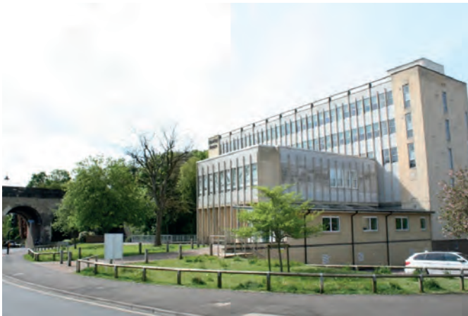
Fig 1.8: The refurbished Bewley House which is set back from the road enabling the whole of the viaduct to be seen.
