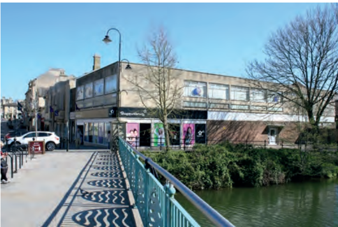
Fig 10.6: No. 1 High Street (Superdrug) is completely at odds with its neighbour and surrounding buildings being flat roofed, having horizontal fenestration and concrete facing, and has a poor relationship with the River.
