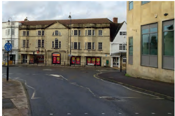
Fig 14.5: The imposing frontage of this former coaching inn is a local landmark. Converted into a supermarket in the 1970s, the character of the frontage has been severely compromised by the brutal truncation of the bays, insertion of plate glass and recessed entrances, and shows a complete lack of respect or understanding for the form and layout of the façade.
