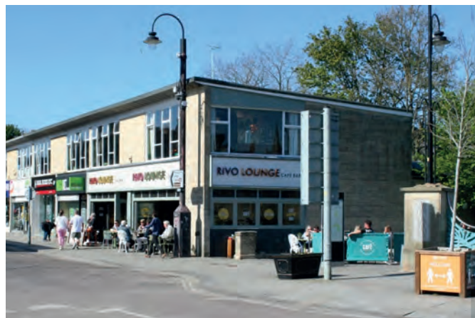
Fig 7.7: Whilst this building has a strong uniform horizontal emphasis at odds with prevailing urban form, the retro styled Rivo Lounge has added an appropriate, and highly popular use.
