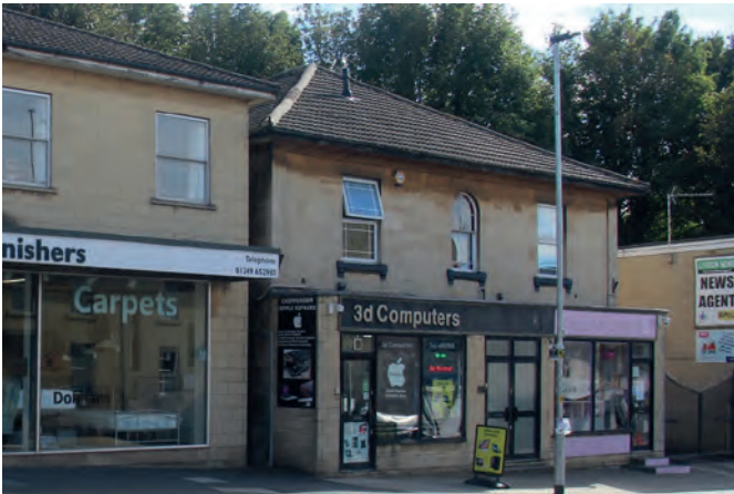
Fig 3.6: Replacement UPVC windows are out of character with most historic buildings, particularly in their obtrusive means of opening compared to sash windows. Compare with the central original window.
