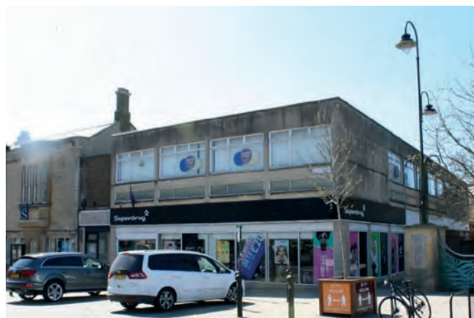
Fig 12.3: The poor architectural and townscape quality of No. 1 High Street is an eyesore in its prominent location and surely warrants its replacement with more suitable high quality replacement.
