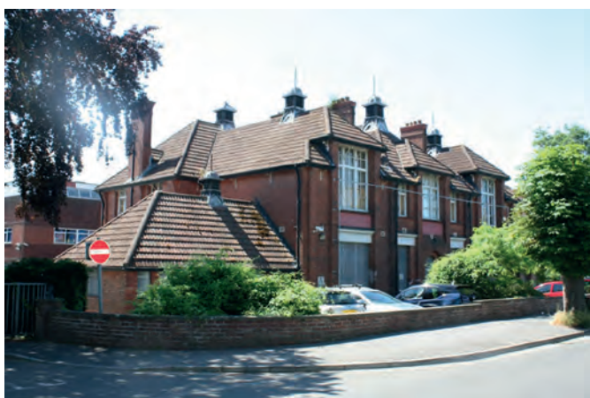
Fig 4.4: The attractive Victorian frontage of the former Technical School building, with the unattractive 1980's extensions behind.
