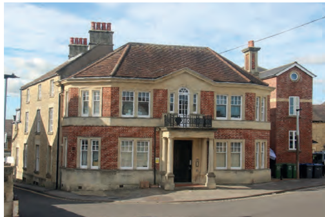
Fig 3.10: The former Georges Railway pub is a notable and attractive landmark at the junction of Old Road and Union Road, particularly when viewed from the footbridge across the railway.
