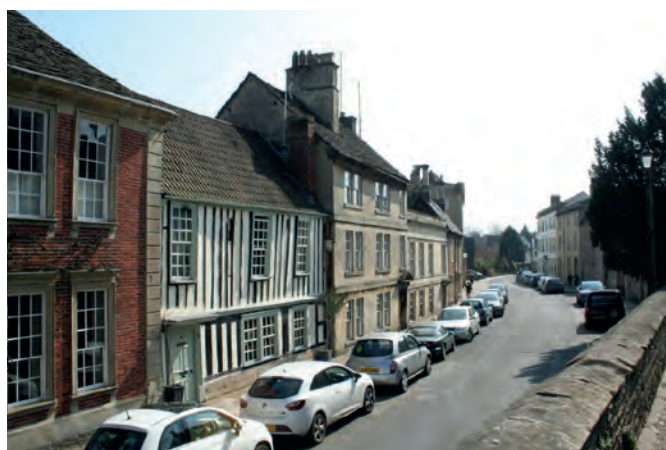
Fig 15.6: The south side of St. Mary Street. Nos. 51 and 50 (to the right) had their timber framed facades replaced with classically styled stone in the early 1800s.
