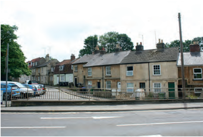
Fig 6.3: The western end of Foghamshire consists of an attractive curving terrace of cottages. These are humble in scale and at odds with the close proximity of fast moving through traffic.
