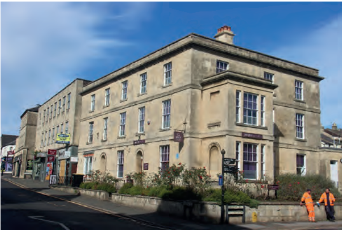
Fig 7.10: Nos. 1-2 is one of the most notable and elegant buildings lining the street. Note how the adjacent Nos. 3-4, although similarly scaled, appears bland and monolithic in appearance. Greater attention to siting, proportion and detail could have produced a far more satisfactory and appealing building.
