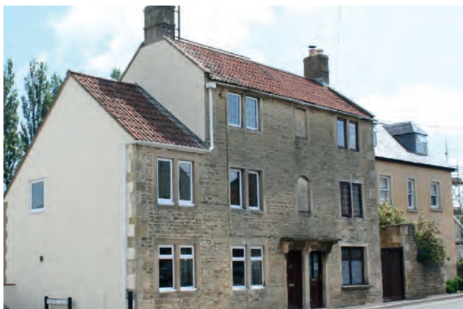
Fig 18.3: This listed building has a well-executed extension but the character of the building is severely compromised by UPVC replacement windows and doors.
