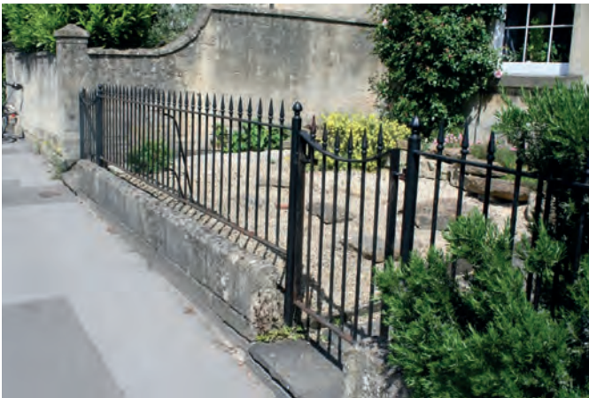
Fig 1.6: Reinstatement of original features such as railings is to be welcomed. However correct guidance is needed to ensure their design and appearance is historically accurate. These railings set behind the wall look odd and defeat the object of having the wall - the wall is for the railings to be set in or on.
