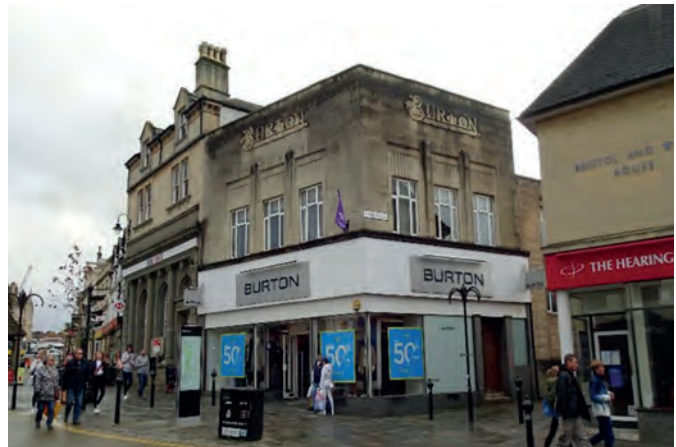
Fig 14.2: The poor shopfront of the former Burton store disguises much of the fine Art Deco building - one of only two in this style in the town centre.
