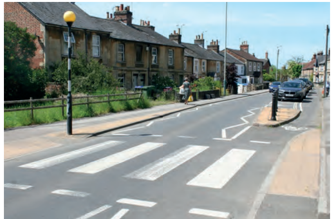
Fig 2.7: Positioning a cycle lane by the kerb has pushed parked cars to a prominent position in the middle of the street and necessitated chicanes and road markings. The whole effect is to add an unnecessary degree of clutter into an otherwise attractive street.
