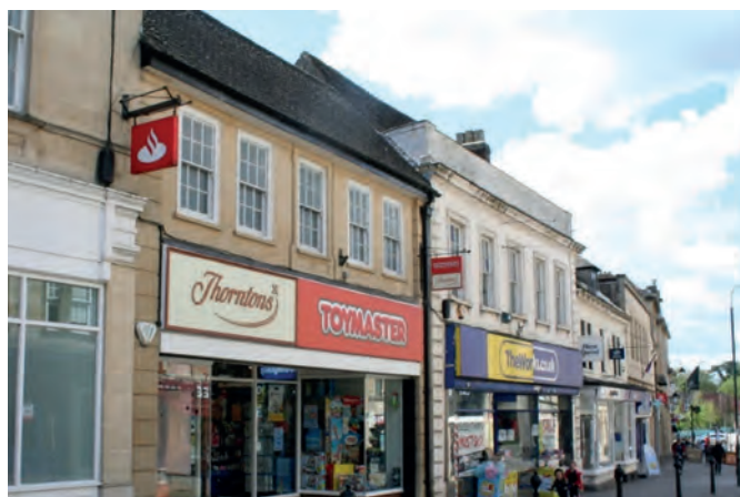
Fig 12.5: This is one example of a number of shopfronts that fail to respect the character of the building of which it forms a part. This is completely out of scale with the building.
