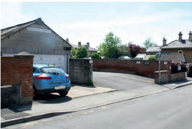
Fig 2.4: The top end of St. Paul Street is less attractive, consisting of unattractive rear entrances to properties on New Road and Park Lane. The frontages are poorly defined and the sense of enclosure and human scale breaks down.
