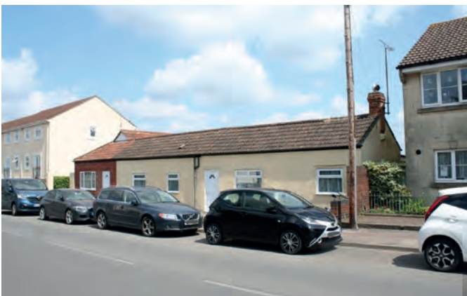
Fig 18.1: This diminutive building is out of scale with surrounding housing and has a poor quality bland frontage. Redevelopment of this site could bring significant townscape enhancements.
