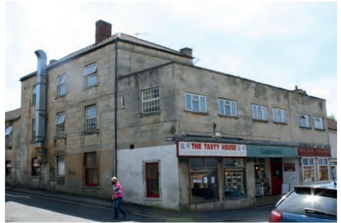
Fig 3.7: The projecting addition to No. 18 is a particularly disruptive element in the building frontage and obscures buildings beyond, when viewed from either direction.
