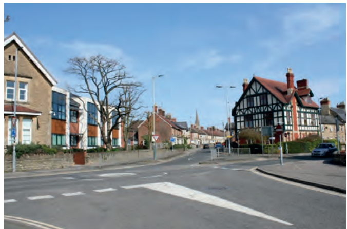
Fig 1.4: The junction between Marshfield Road, Park Lane and Audley Road. To the left is the elegant, recently built, premises of the Probation Service, and to the right West End House which was converted into residential in 1990. Most noteworthy is the over dominant highway design which makes crossing by foot or bicycle unpleasant and extremely challenging.
