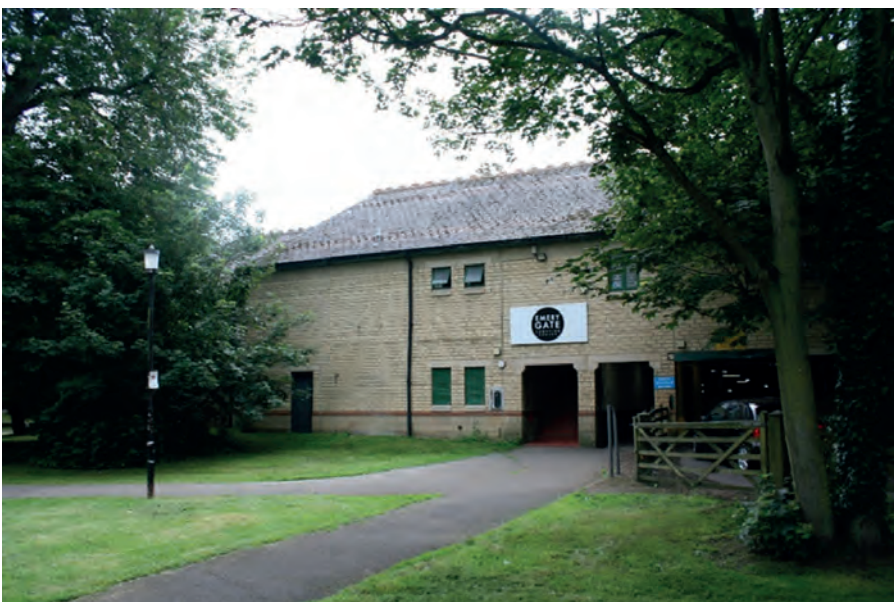
Fig 11.4: The unattractive blank elevation of the shopping centre is an intrusive feature along much of the south side of the island park.
