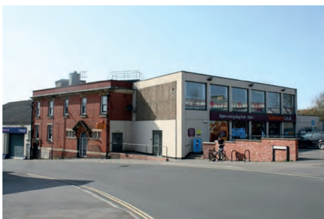
Fig 8.12: The pleasant former post office building was one of the first to be built along the street. The 1960's rear extension has been elegantly converted into a Sainsbury's store.
