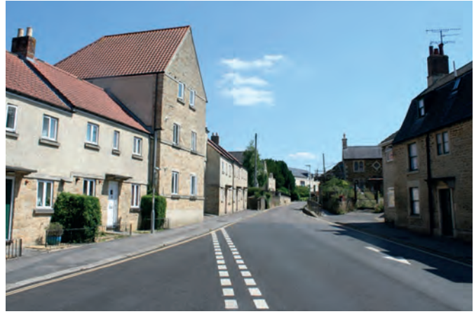
Fig 13.7: These newer houses and flats do little to enhance the Conservation Area. The high gable is an overbearing and inappropriate feature and details such as the diminutive railing design and window units with cills that duplicate the stone cills below are examples of poor attention to detail. The roof tiles are out of place too.
