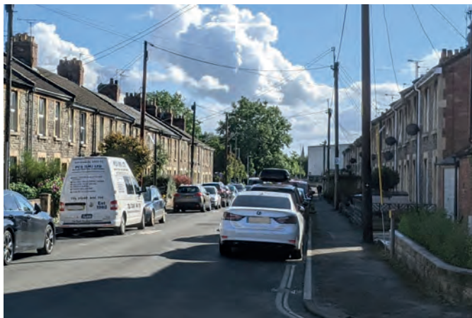
Fig 5.1: Tugela Road is a typically urban street of solid terraced houses but the overhead wirescape is a notably intrusive feature.
