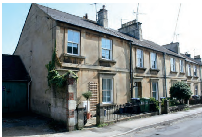
Fig 2.5: Houses near the top of St Paul Street where some of the correct sash windows and railings were restored following a past campaign by Chippenham Civic Society.
