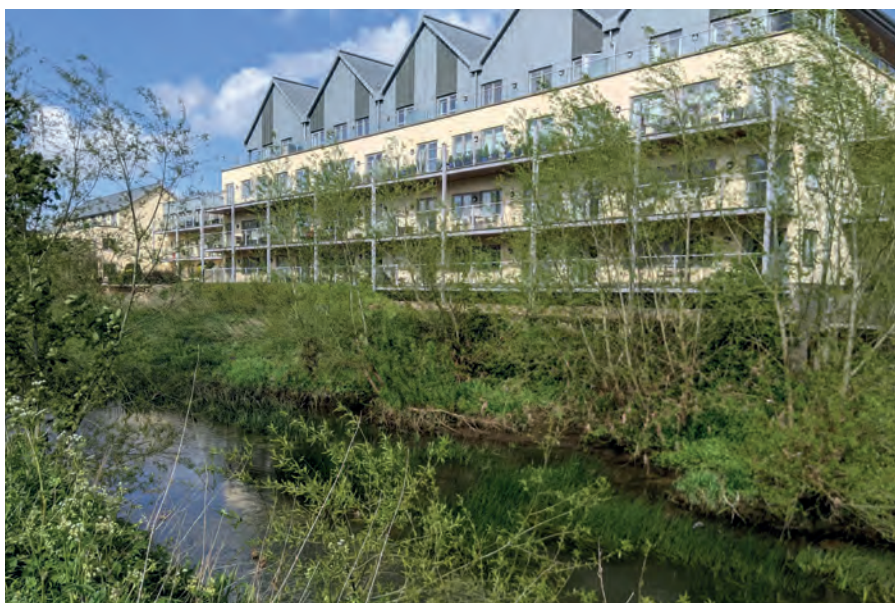
Fig 16.2: Attractive rear elevation of Bowles Court
